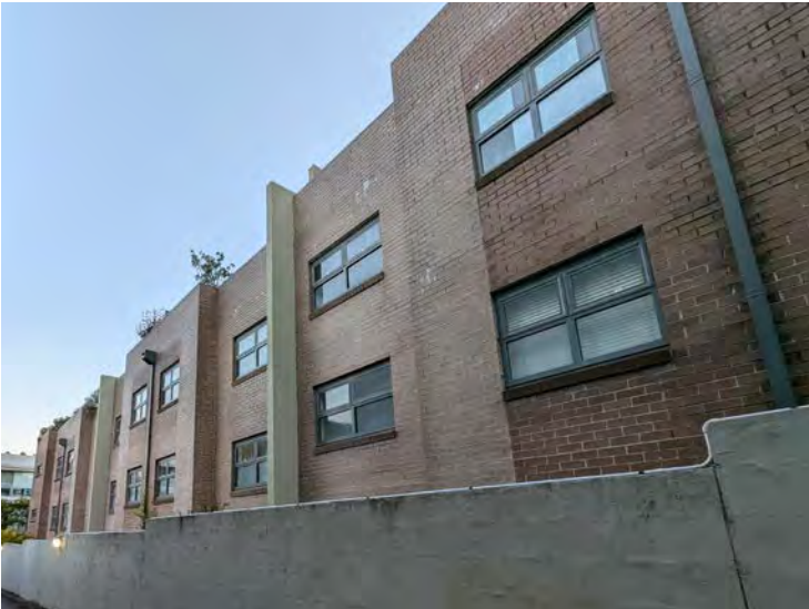
Rear of 15-41 Cornwallis Street
